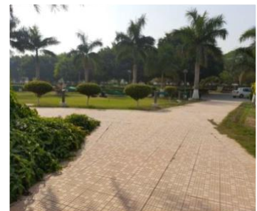
AAC PAVER BLOCKS IN PARKING AREA
